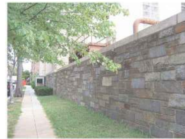
3. 29th Street (West Wall) - Looking North
