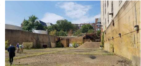
10. Tower East Wall
