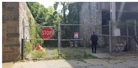
5. West Wall - South
