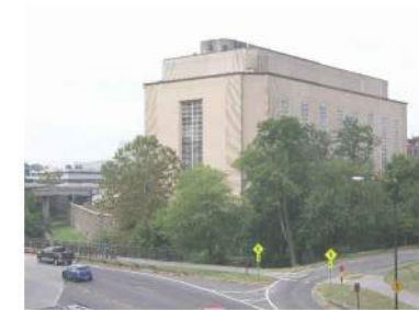
9. View from Highway (NE)
