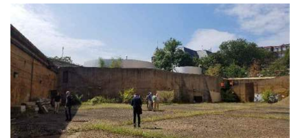
11. Exist. South Wall
