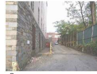
8. Tower East Wall
